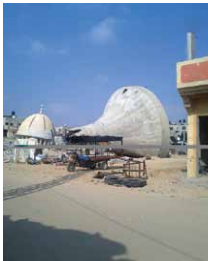
Destroyed water tower and mosque, Khuza'a. Photo by AV, 12 Nov 2014
